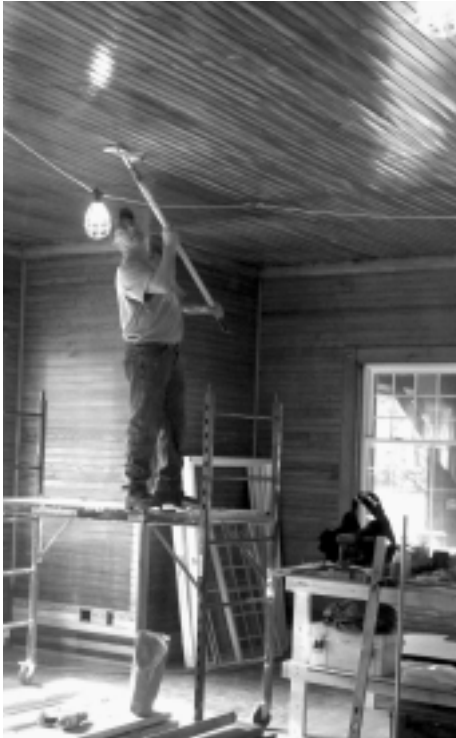
Ron Johnson sands the gloss finish off the wood to prepare it for refinishing with a satin finish sealer.
